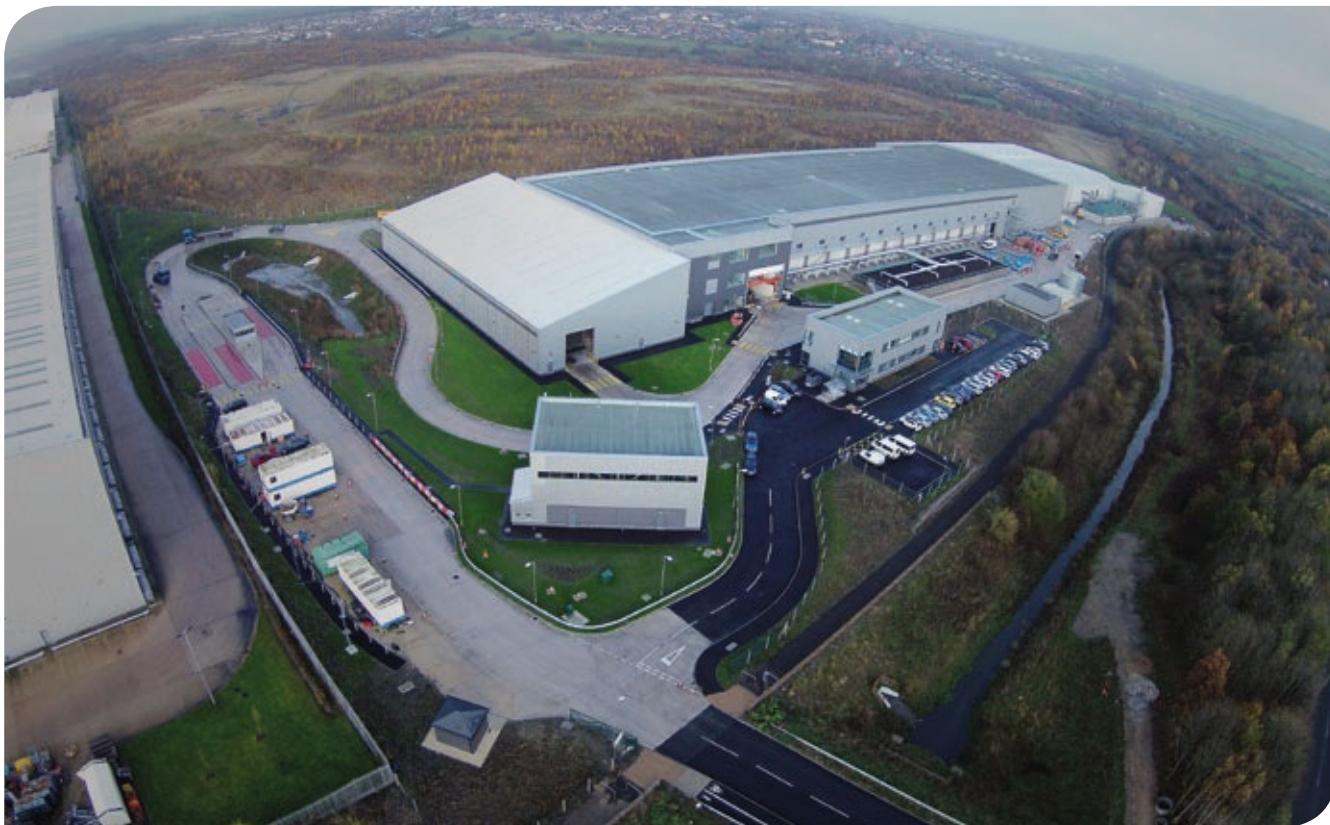
Our new BDR facility in Rotherham, UK
